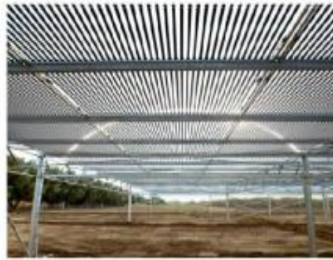
Example of innovative PV using cylindrical modules (Solyndra inc.) and Poinsettia cultivation
