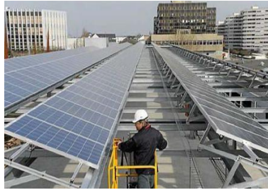
Farms, industrial, service sector buildings
