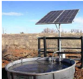
Solar water pumping
